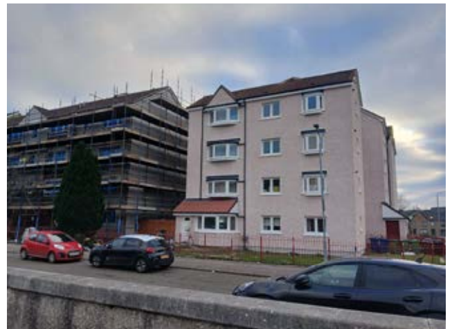
Recent External Wall Insulation work in progress
