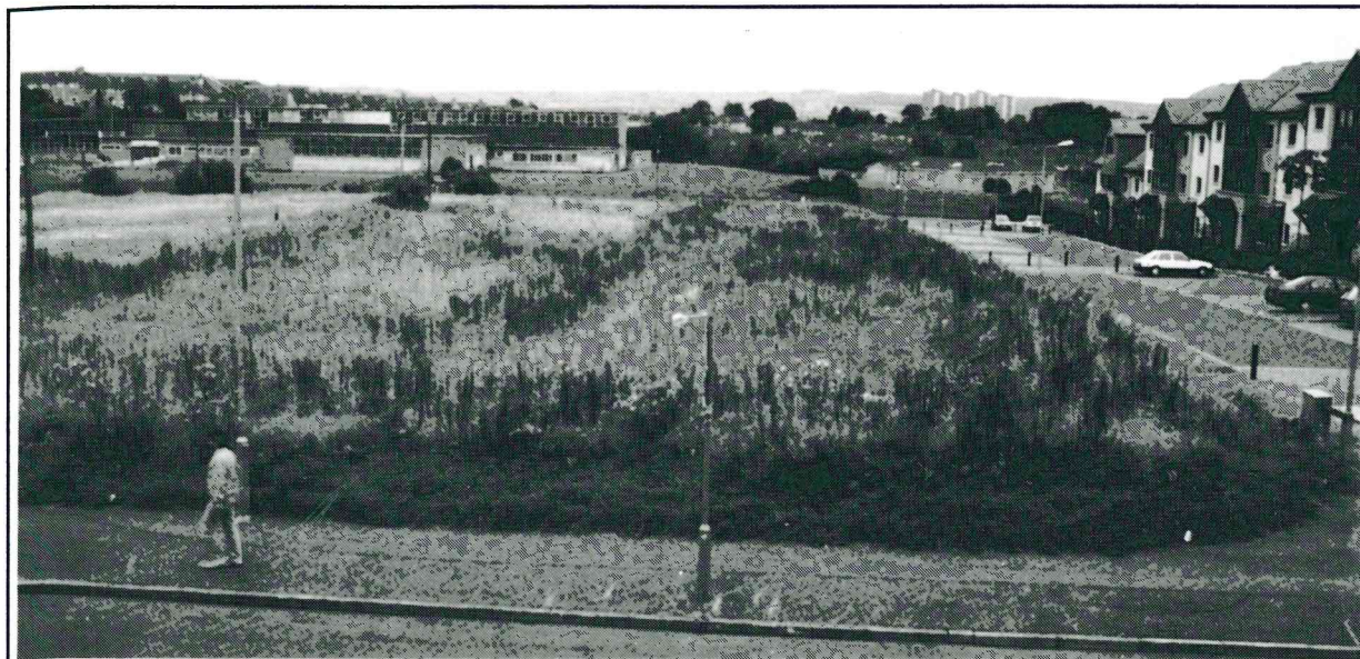
Cleared site at Burnett Road/Barlanark Place
